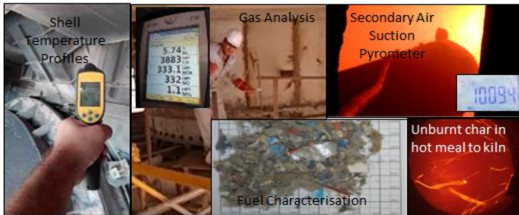
Figure 4: Site survey measurement and data collection.
