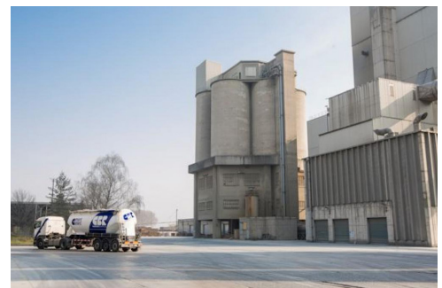
CBR Cimenteries - Heidelberg Group, Antoing, Belgium.
